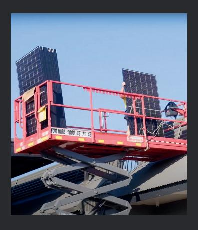
Similarly, at McDonald's Eagle Vale, we installed Trina 440 watt S+ solar panels, each featuring a SolarEdge optimiser. These optimisers allow the panels to operate independently in shaded conditions, significantly boosting overall energy yield. The SolarEdge three-phase commercial inverter we installed ensures optimal power conversion and integrates with the optimisers for real-time monitoring, helping McDonald's Eagle Vale reduce energy costs and enhance sustainability.
